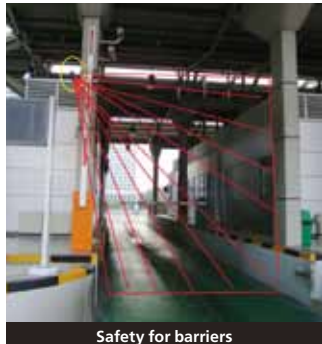
Safety for barriers
